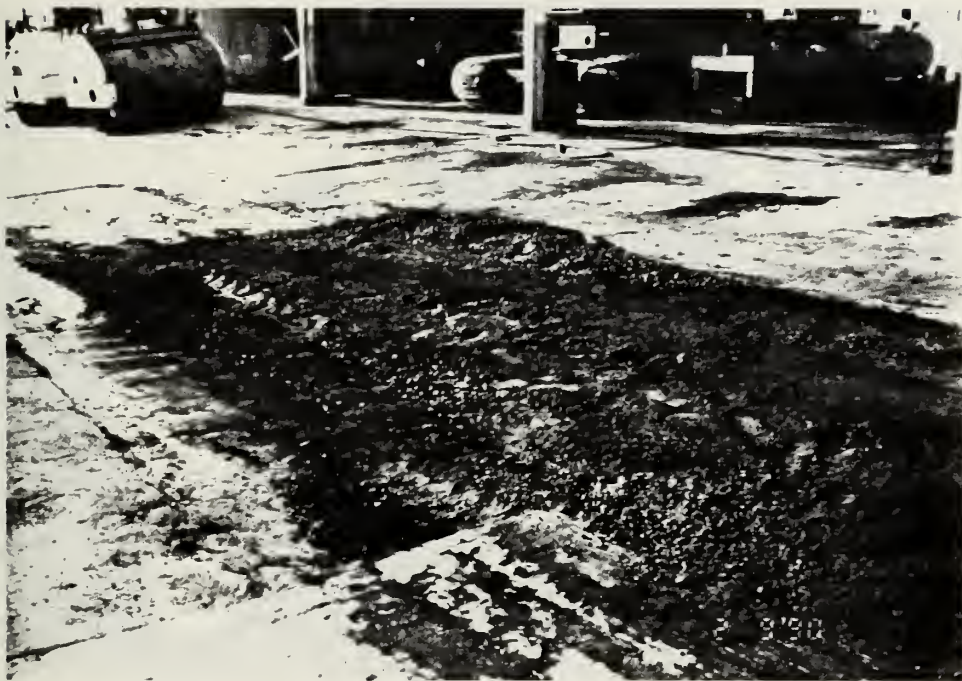
Figure 5.4 Mixed, Uncompacted Slab
